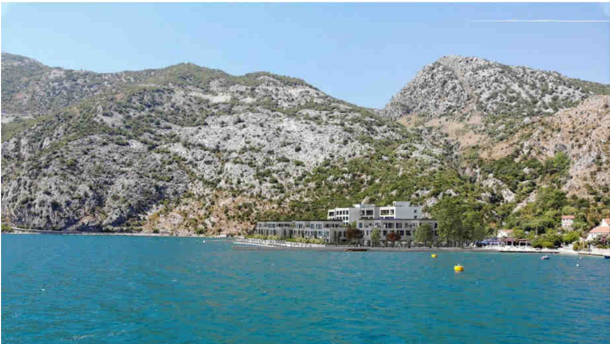
Fig. 4: View from the south-east across the bay, as existing and as proposed.
